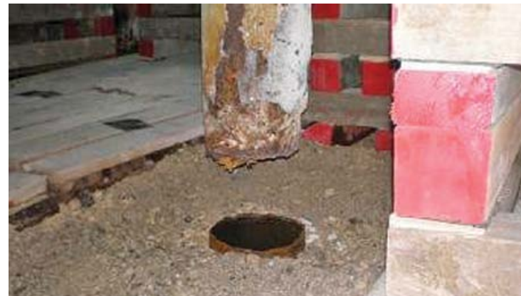
Disconnection of pipe.
