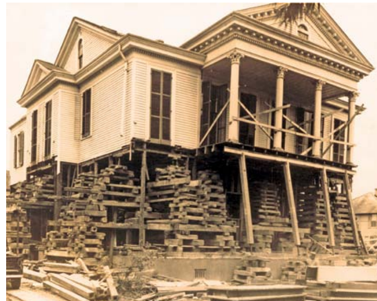
House on wooden cribbing with ground story removed.
