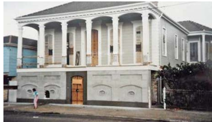
TOP: Early-1980s view of steel used to support a house during elevation project on Rampart Street.
