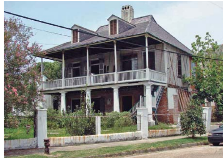
Same dwelling under restoration following Hurricane Katrina.
