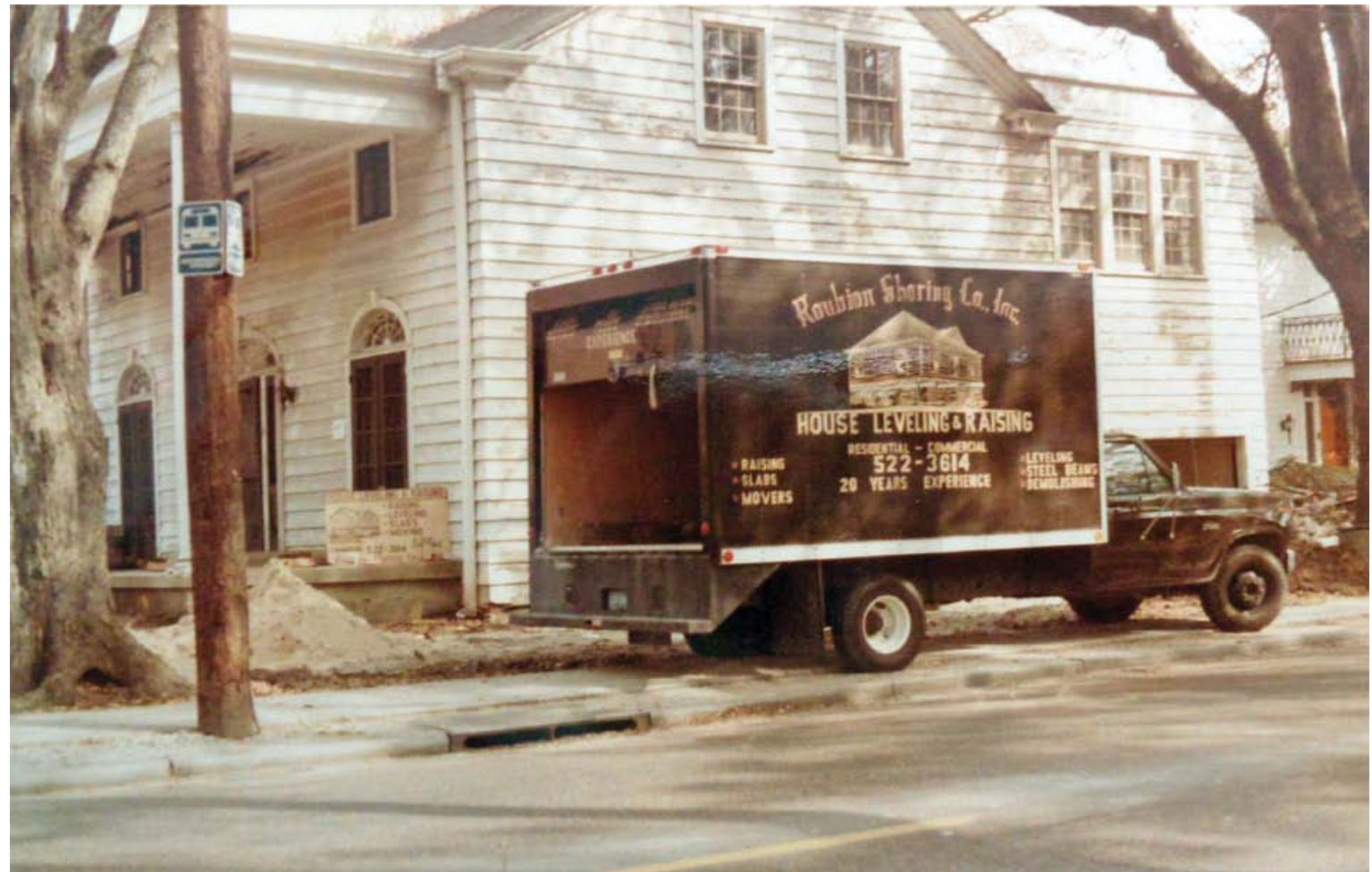
Site photo from Roubion Shoring Company, Inc., ca. 1970s.
