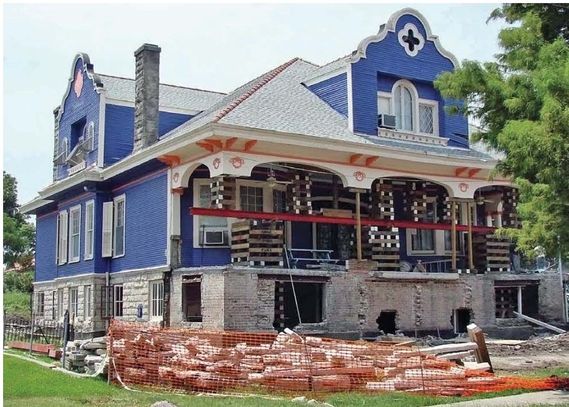
Raised Basement house at 1219 North Lopez Street undergoing restoration in the aftermath of Hurricane Katrina.
