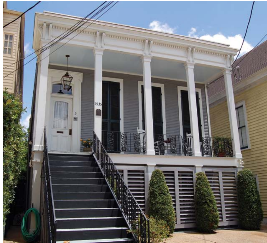
Façade of 1535 Seventh Street, at left, with modern louvers shading basement.
