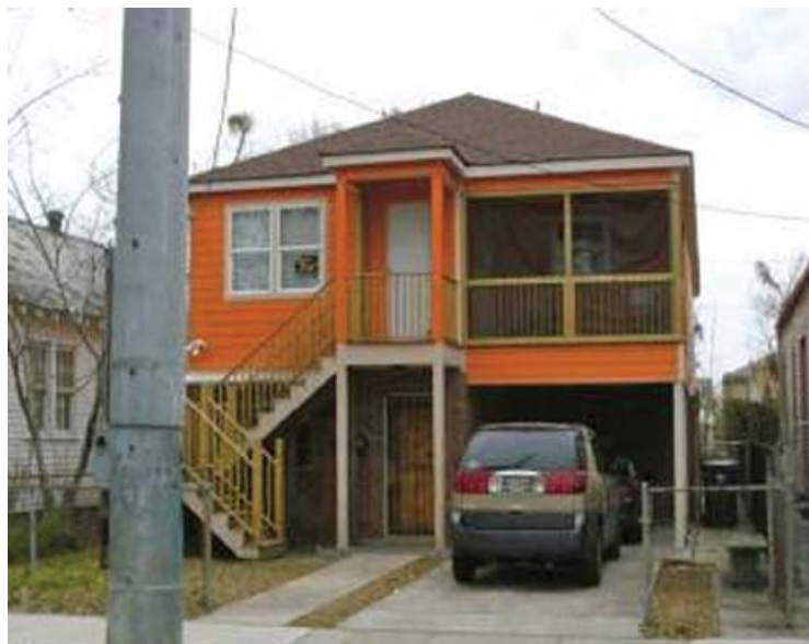
Before-and-after views of a second-story conversion.
