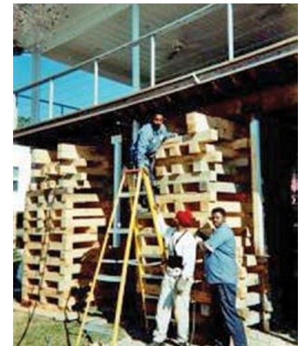
Cribbing assembled by Abry Bros. crew, early 1990s.
