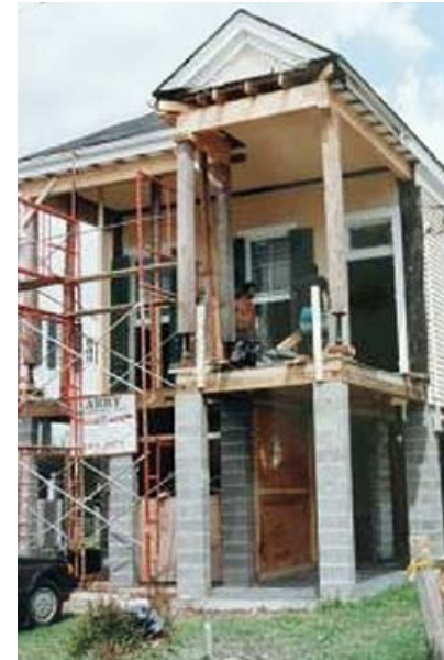
RIGHT: Samuels-Epstein house, during renovation and elevation.
