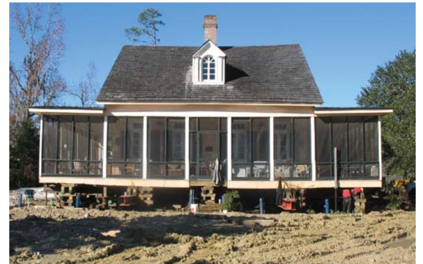
BELOW: Francois Cousin House in October 2009 before elevation on piers and construction of berm, at left, and after, at right.
