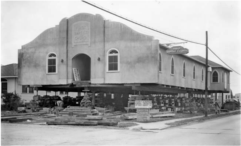
First Baptist Church, Gretna, being elevated by Norton Shoring, ca. 1940s.
