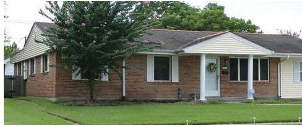
Slab elevation, before-and-after views.
