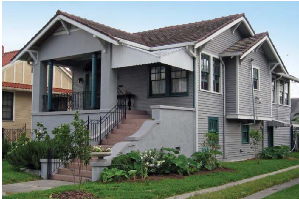
TOP: Raised Basement bungalow at 4045 Fairmont Street, Edgewood Park.
