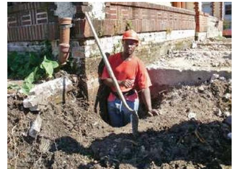
Excavation at Rosa Keller Public Library, Broadmoor neighborhood, 2011.
