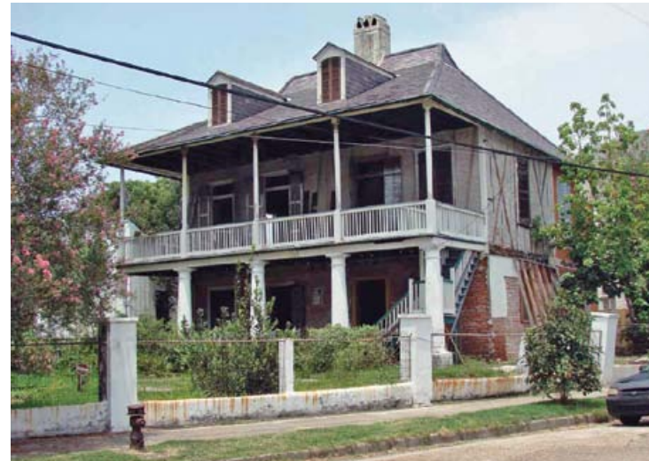
Same dwelling under restoration following Hurricane Katrina.
