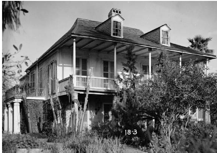
Raised Creole Cottage-type dwelling at 1300 Moss Street in New Orleans in 1934.
