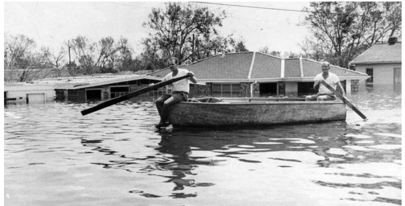
North Claiborne Avenue after Hurricane Betsy, September 1965.
