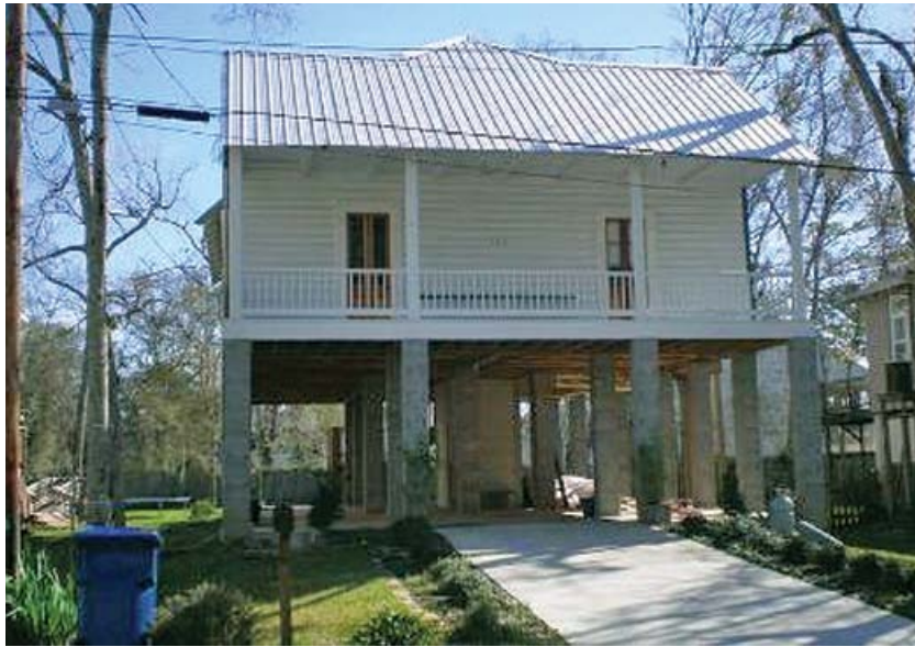
Creole Cottage-style house in Mandeville elevated on cribs (top) and following elevation.
