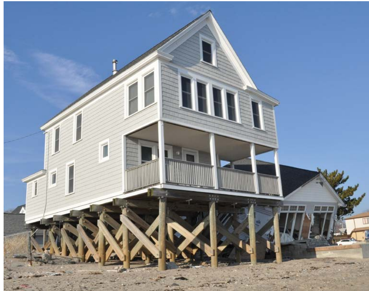
Example of a building on pilings.
